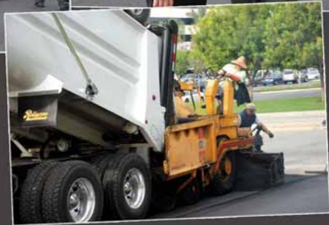
its viscosity until the material has cooled. The foam then collapses and the bitumen behaves as a normal binder. They say water and oil don't mix which is true, but it does create a foaming action, that in turn reduces the viscosity of the binder, allowing for sufficient coating of the aggregates, while maintaining good workability and durability.
